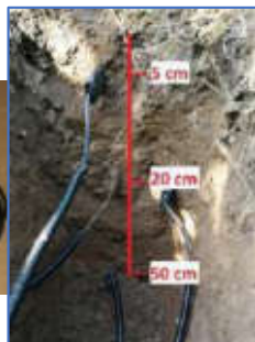
53 clusters for soil moisture monitoring equipped with 318 TDT sensors
